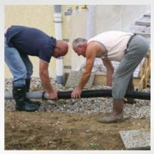
The delivery line is quickly laid and routed. A total of 45 m of delivery hoses and 45 m of delivery line are carried with the pump.
