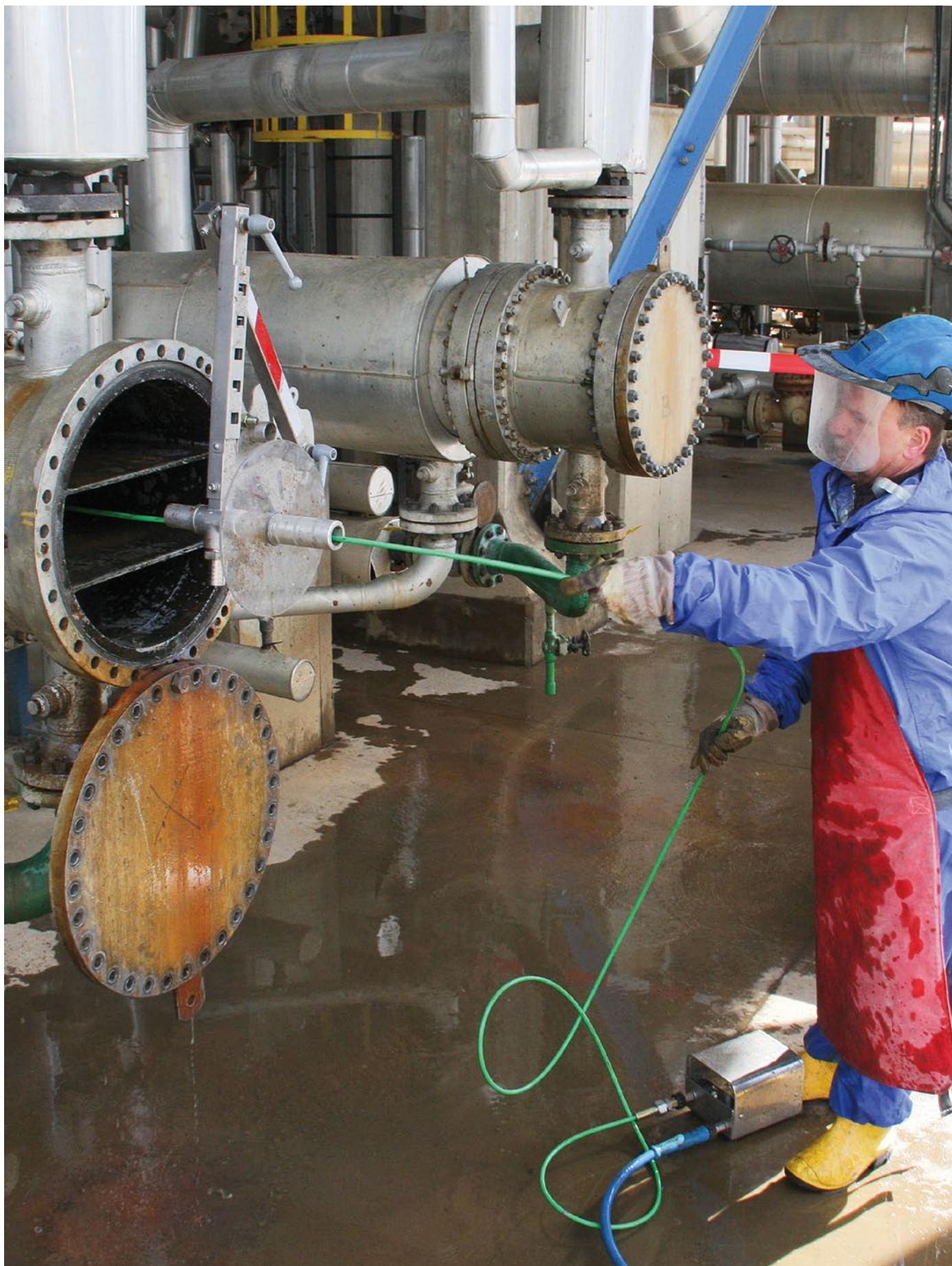
Cleaning heat exchangers
