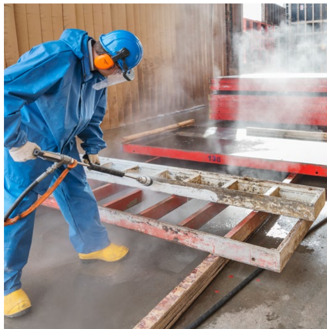
Cleaning shuttering
